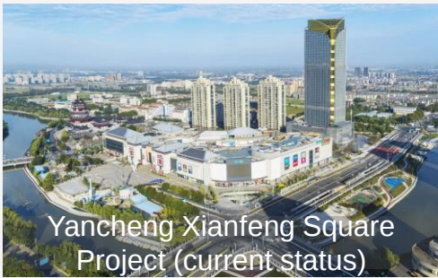
Operating Projects under Renovation
